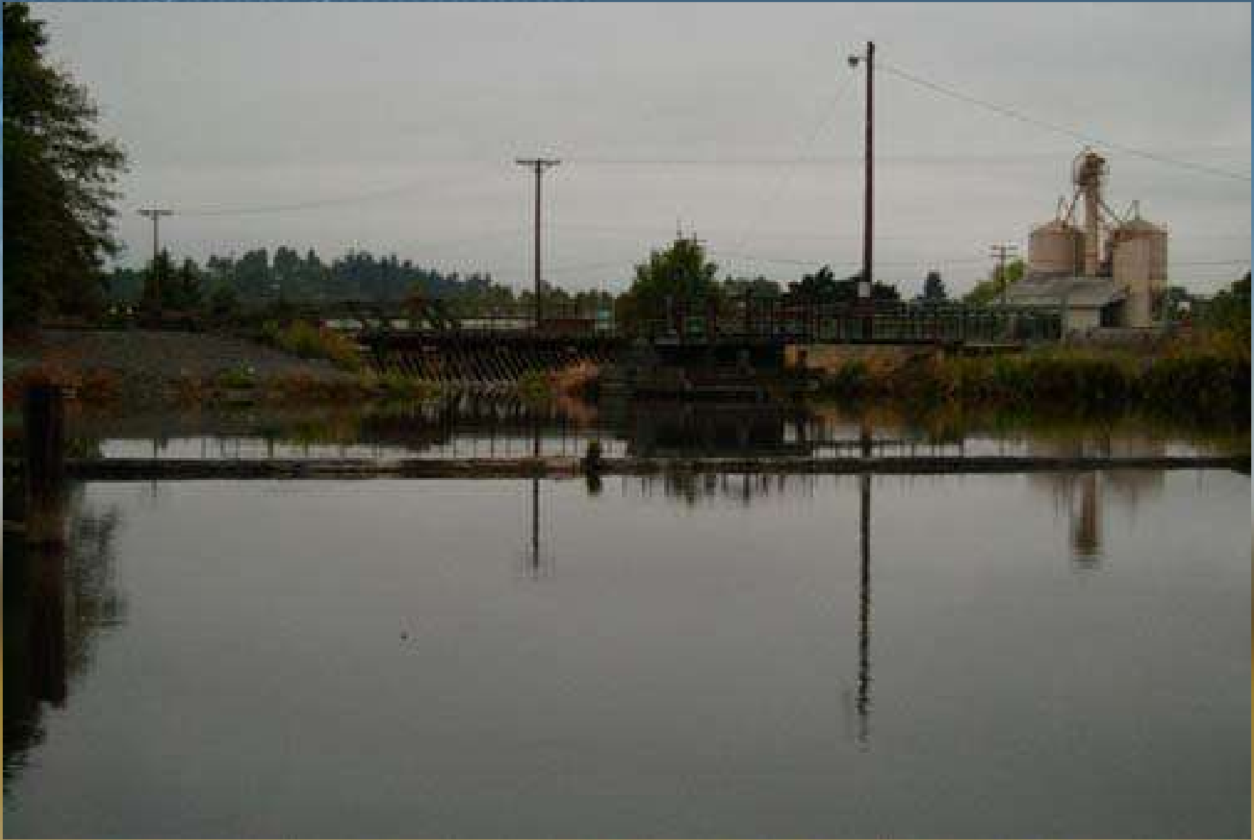
Springfield Millrace Dam
