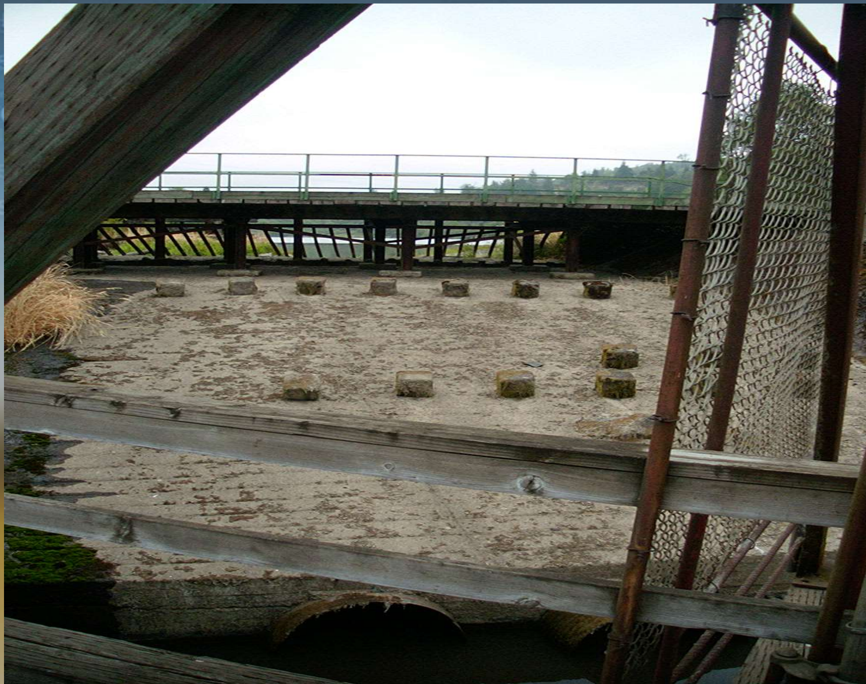
Springfield Millrace Dam
