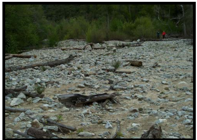
Figure 5. Accumulated debris in upper reservoir
