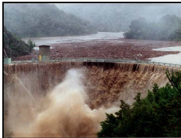
Figure 3. San Clemente Dam during flooding
