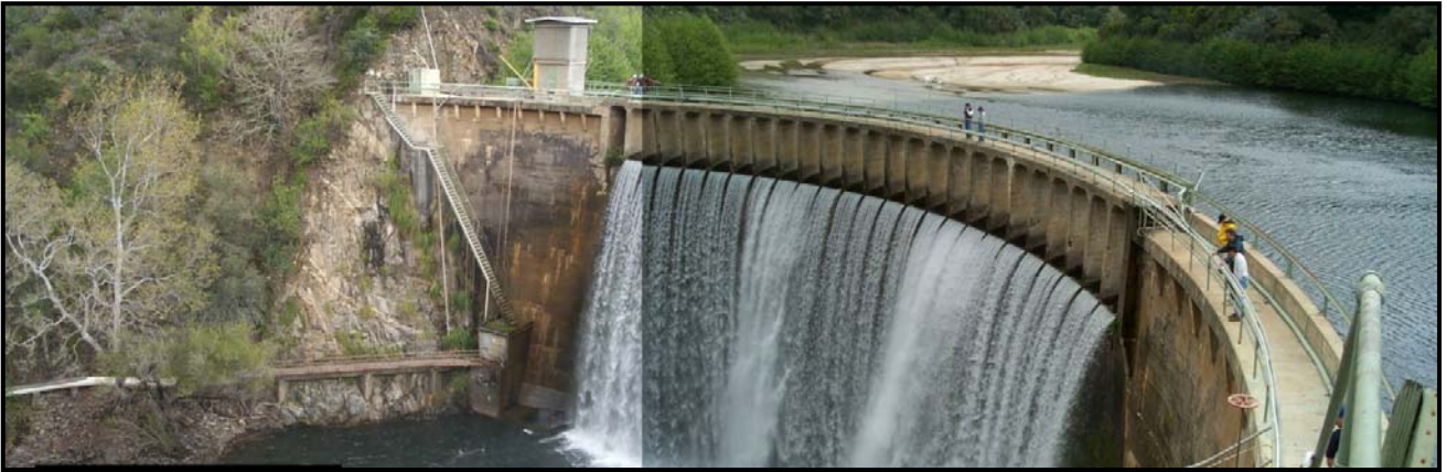
Figure 4. San Clemente Dam and Reservoir
