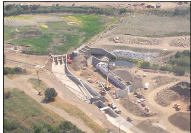
Figure 9. Robles Fish Ladder under Construction
