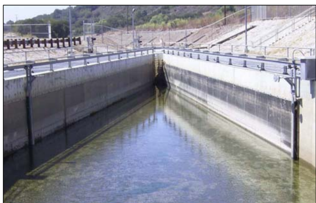
Figure 11. Fish screen and cleaning brushes
