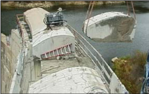
Figure 7. Concrete removal in 2000
